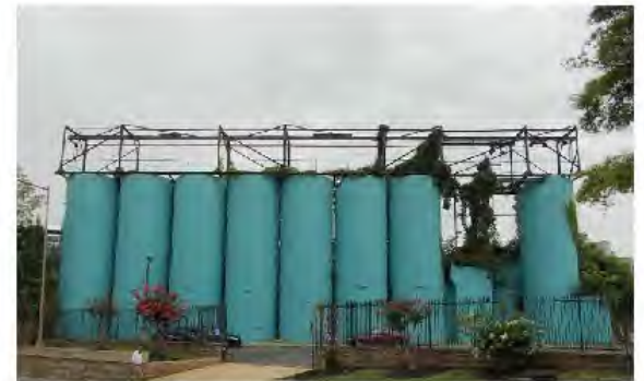
J. Silos on Rhode Island Ave.
