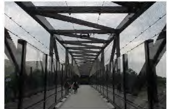
F. Metro Bridge
